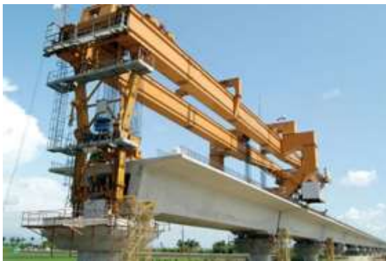
Precast Deck slab launching
